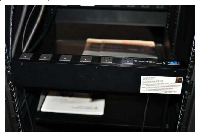
The T10X has a total of ten outlets - six mounted on the face panel of the unit, and another four mounted on the back panel. Like the PWRI-PRO, the T10X uses their best X3 MOV protection technology for maximum protection from surges and spikes.
